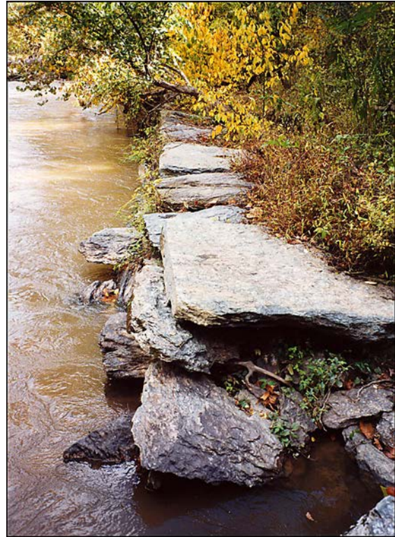
Wall along Virginia shore for Seneca sluice (D. Guzy)
